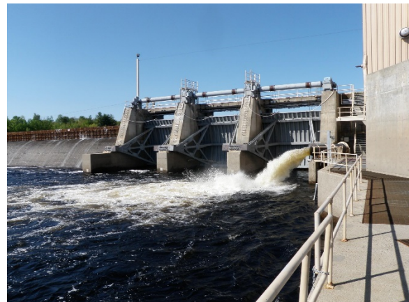
West Enfield Dam in Maine's Penobscot River. Photo Credit: Zydlewski Laboratory.
